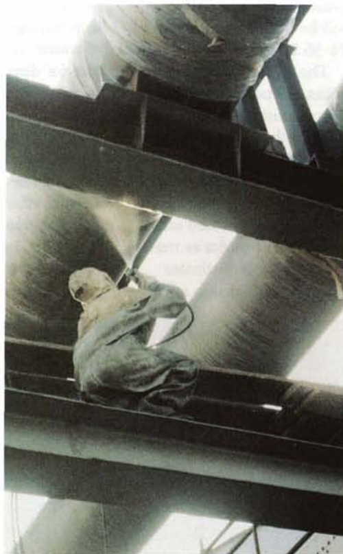
In Saudi Arabia, a worker sprays Chartek Fireproofing on structural parts of a crude oil processing plant. The long life fireproofing material is a spinoff from the heat shield that brought returning Apollo astronauts safely through temperatures as high as 5,000 degrees.
